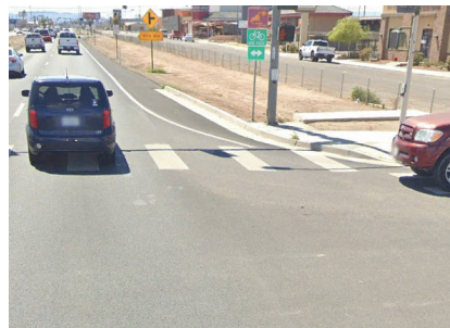
Photo 3: Existing crossing with missing sidewalk
