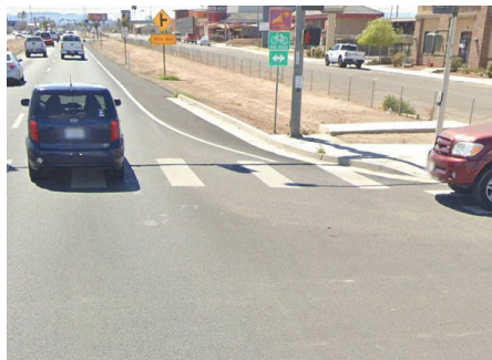
Photo 3: Existing crossing with missing sidewalk
