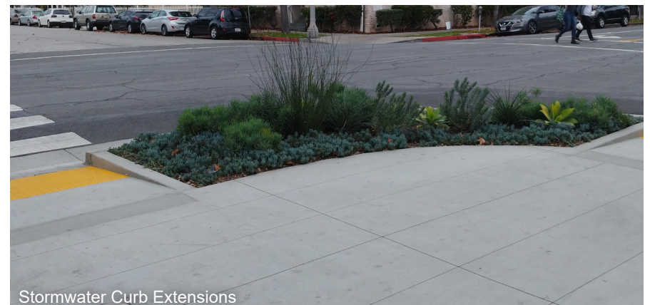
Stormwater Curb Extensions
