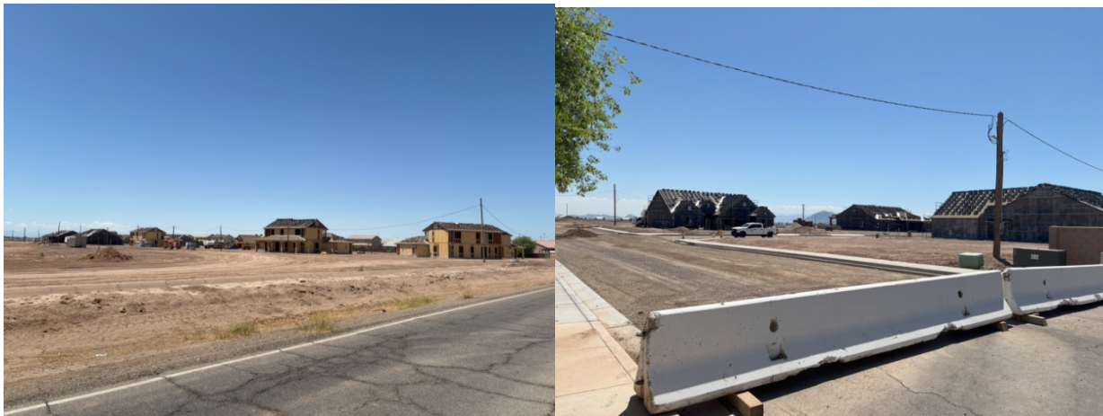
Exhibit B.2 & B.3 Photo of construction on Manzanita Drive (Unit 2B)
