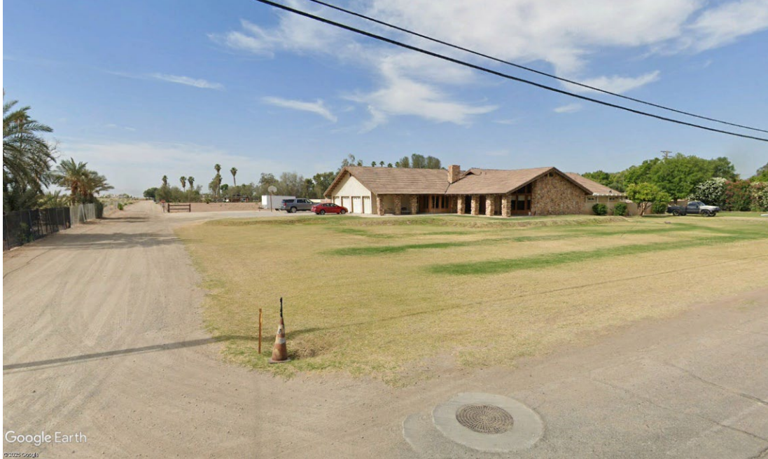
View of property along Main Street frontage looking southwest
