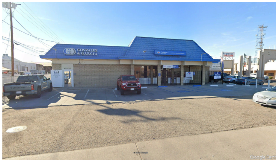
Photo of project site, viewing east
