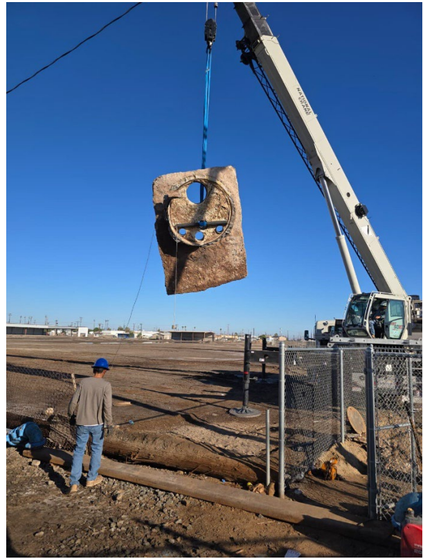
Removal of top failed slab/lid
