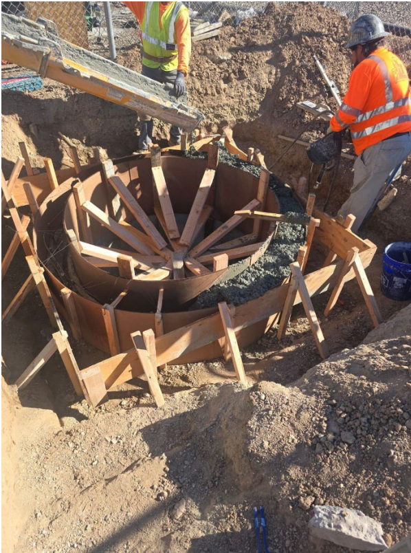
Repair of top wet well wall
