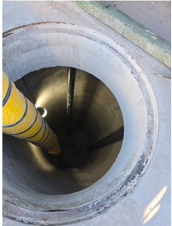
Finished repaired wet well walls
