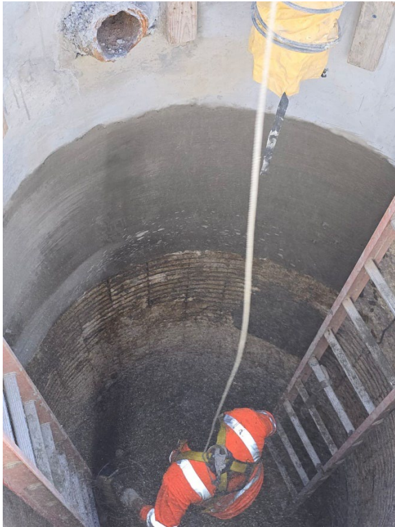
Cleaning and preparation of wet well walls
