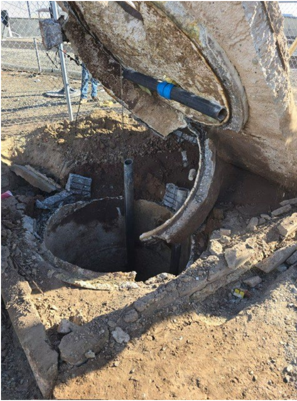
Demolition of the top failed slab
