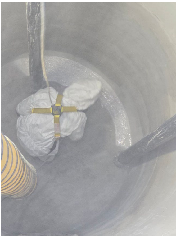
Wet well wall protective coating spray
