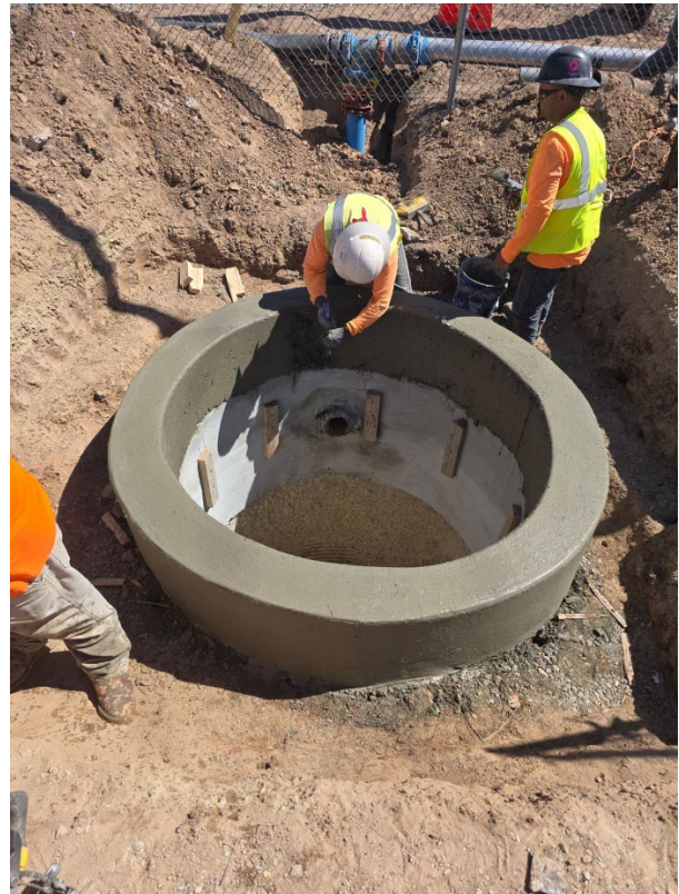
Repair of top wet well wall
