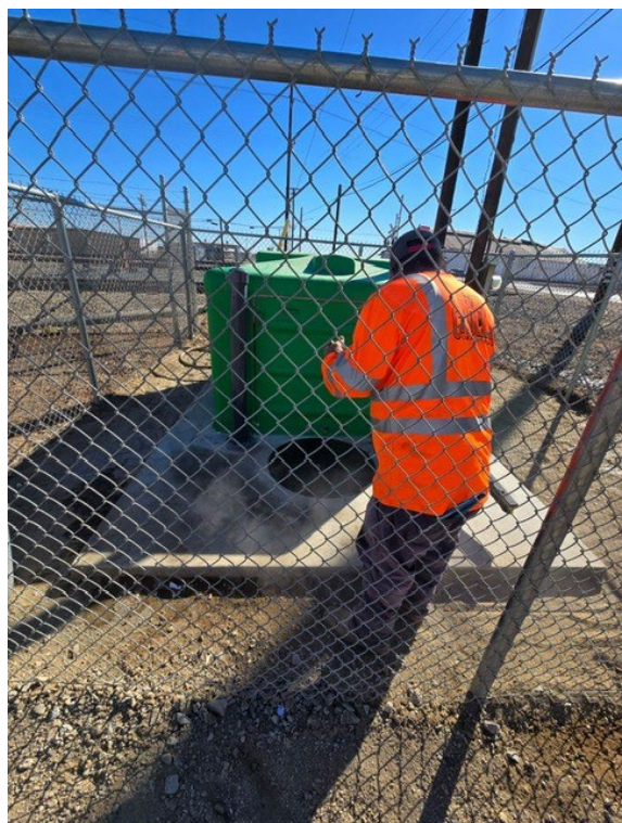
Final inspection after pump is installed over well
