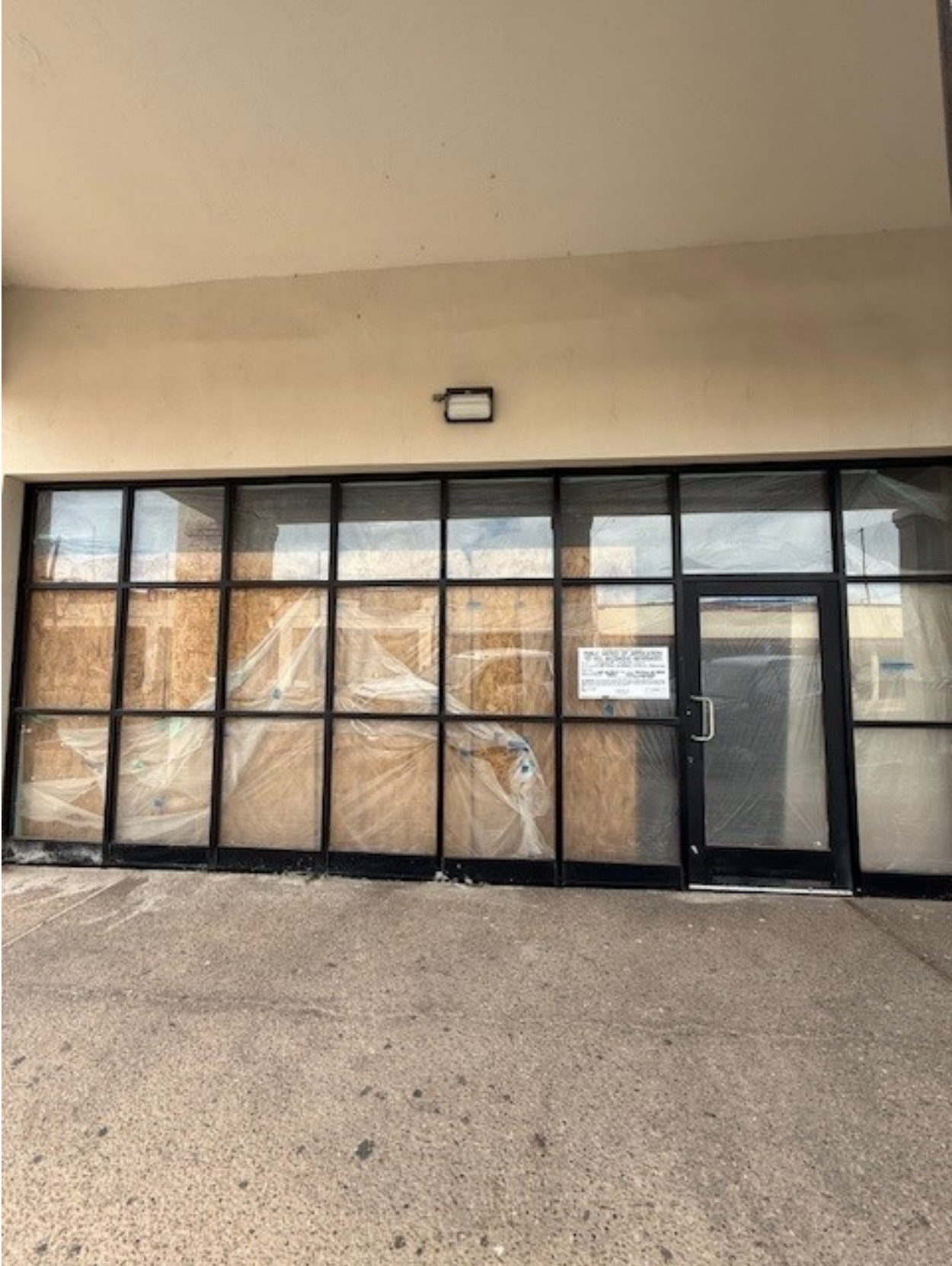
Front of Building
