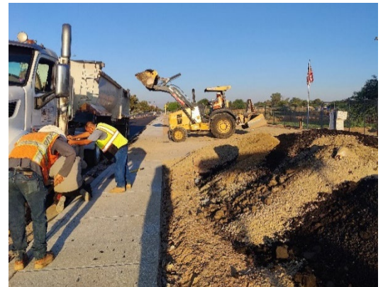
Construction services included full-time construction inspection, daily and weekly reporting to the City and weekly safety and progress meetings with the GC.
