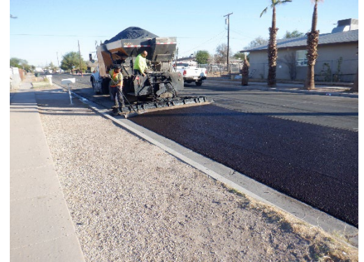
Paving and Type II slurry operations for 2020 Street Maintenance and Rehabilitation Improvements Project
