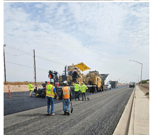
The project involved grinding of existing asphalt concrete pavement and overlaying with ARHM-GG on ARAM over Leveling Course.
