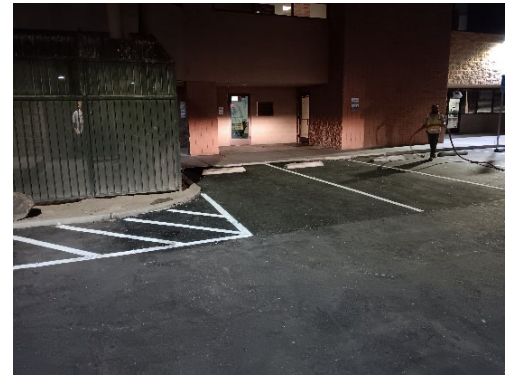
Nicklaus provided on-site inspections and provided a full-time on-site construction inspector and construction manager during the construction activities.
