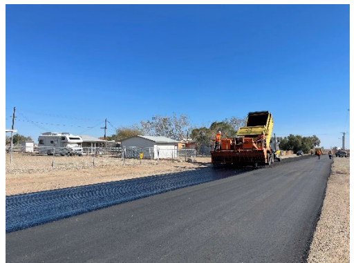
Paving and slurry seal operations at Bombay Beach Townsite.
