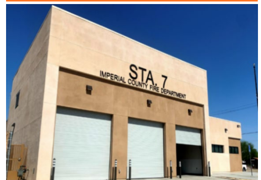
The project consisted of the demolition of the existing County of Imperial Fire Station followed by the construction of a new 7,555 sf County Public Safety Facility.
