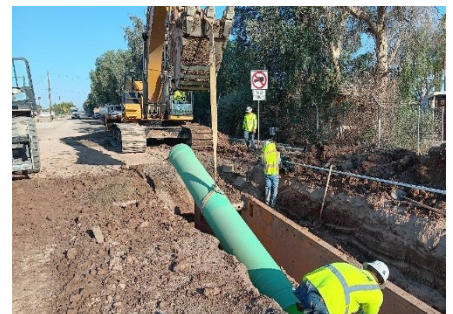
The project involved the construction of a new pump station, along with approx. 4,700 linear feet of gravity sewer main and 2,000 linear feet of sewer force main.
