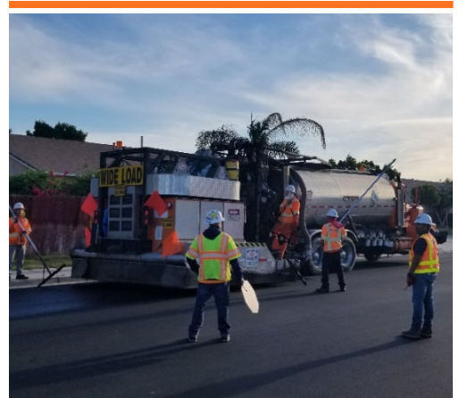
The size of road improvements covered approximately 62,000 square yards. All the work for the project followed the Caltrans Standard Specifications, the project specifications, and the special provisions.
