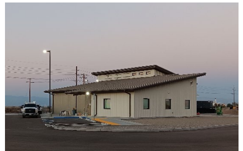
Seeley Public Safety Facility nearing complete build out.
