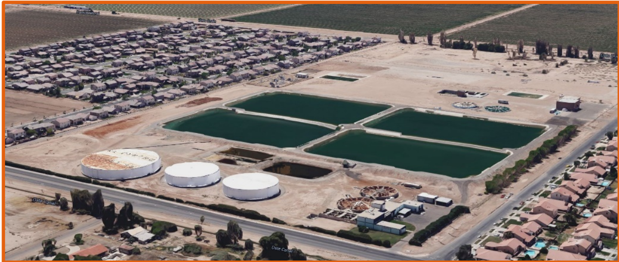
Photo 3-1: El Centro Water Treatment Plant
