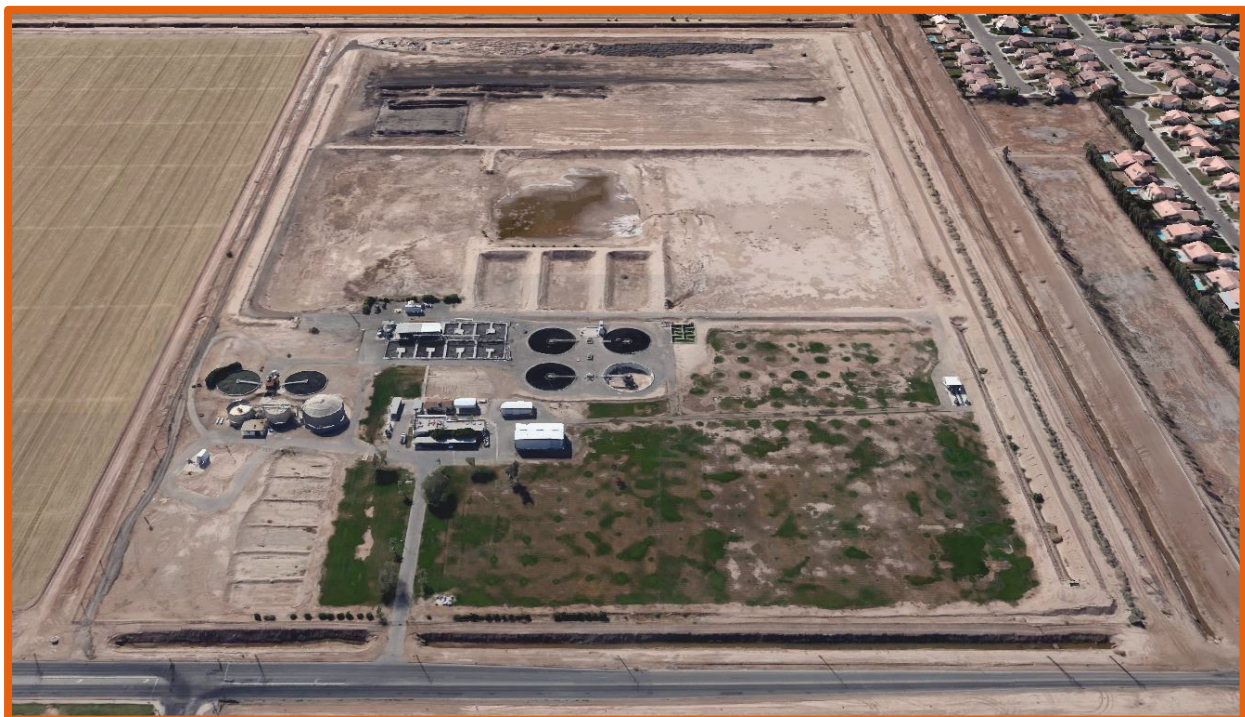
Photo 6-1: El Centro Wastewater Treatment Plant
