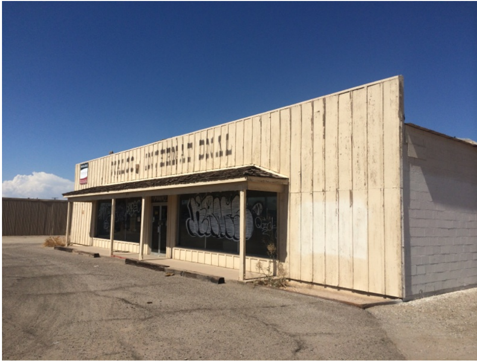
View of the façade of the existing building at the project site.
