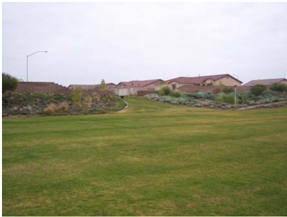
Sample Retention Basin Bottom with Grass
