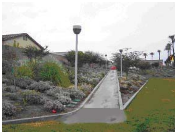
Sample ADA Ramp and Landing
