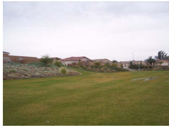
Sample Retention Basin Bottom with Grass
